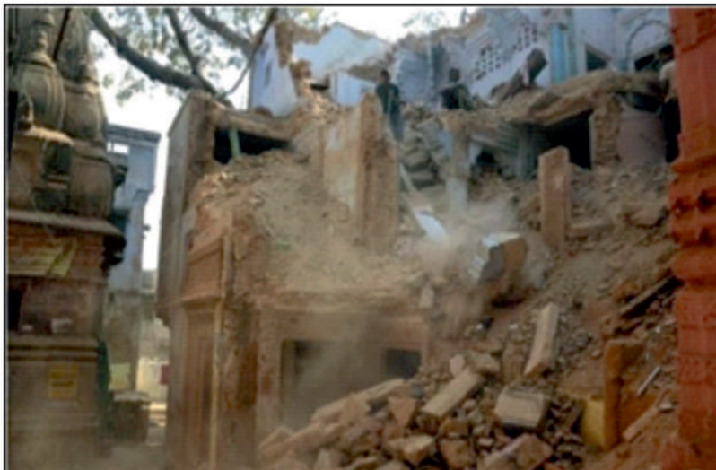
Photo:2 - Demolition Work During Development of Kashi Vishwanath Corridor
